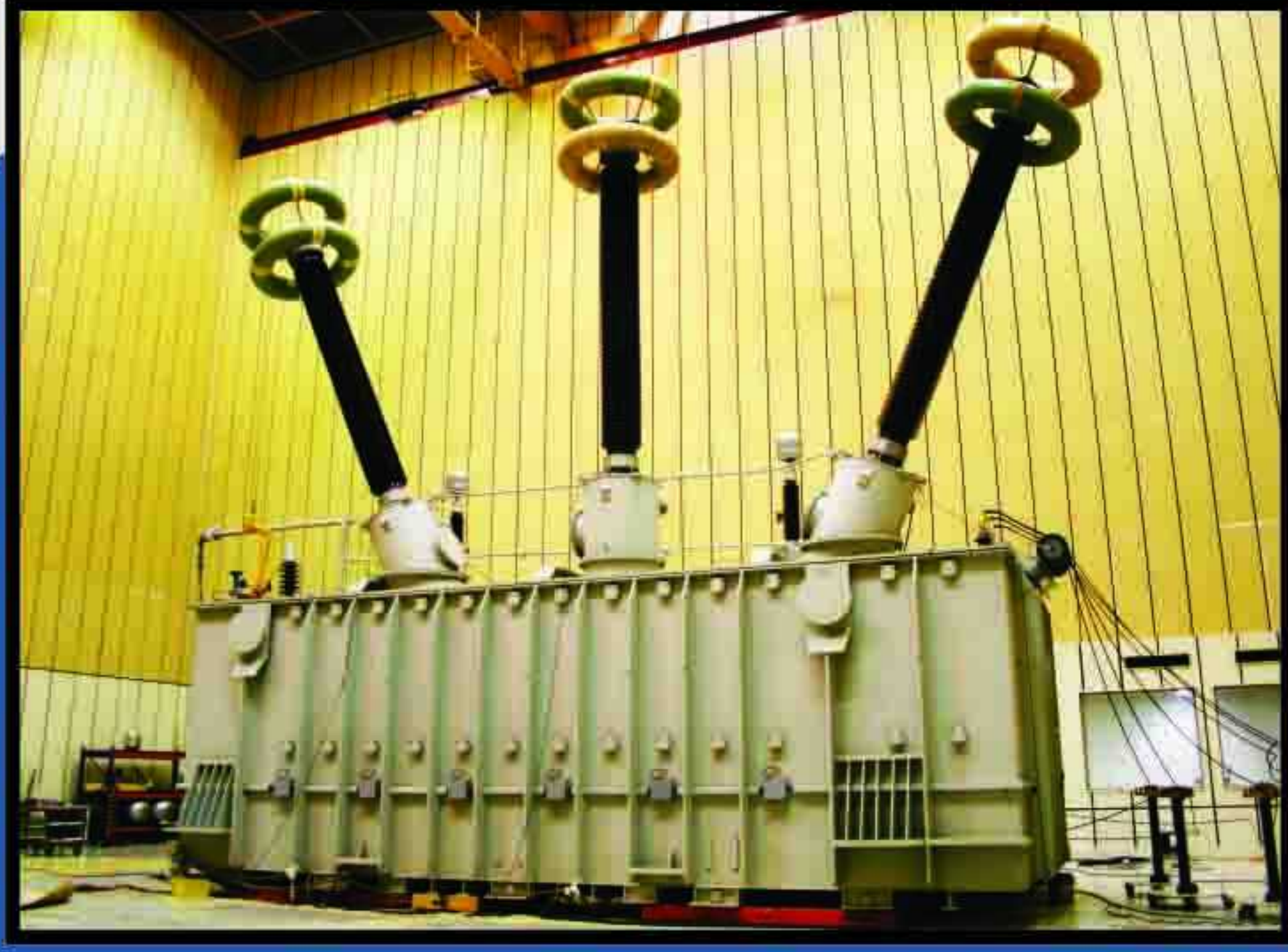
Power Transformer - Neiriz 200 MVA - 400 / 66 / 20 kV
