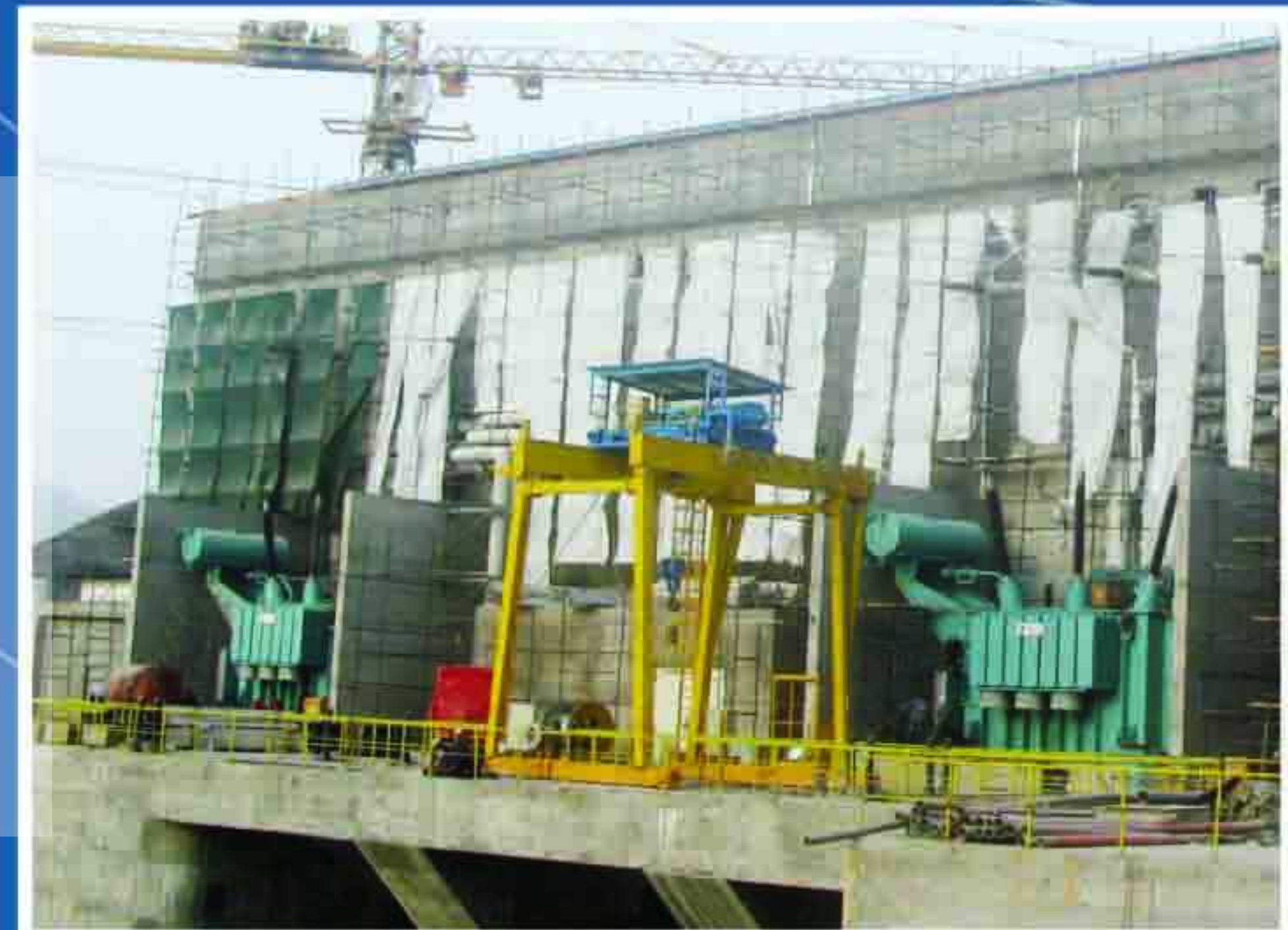
Sangtuda Power Plant - Tajikistan 125 MVA - 230 / 13.8 kV
