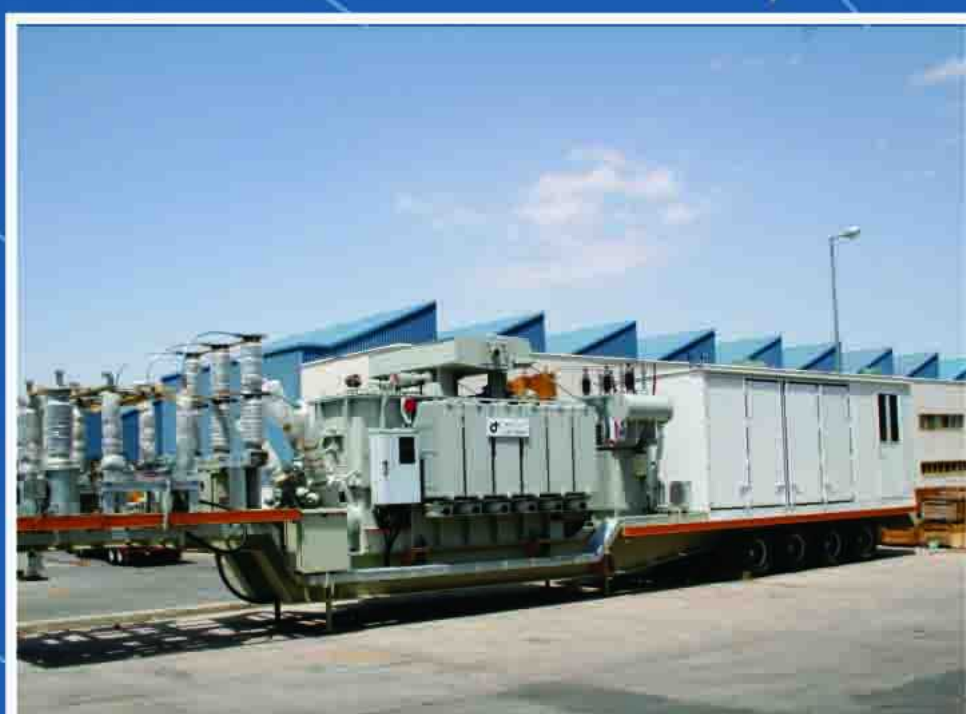
Mobile Transformer - Iraq 25 MVA - 132 / 11.5 kV
