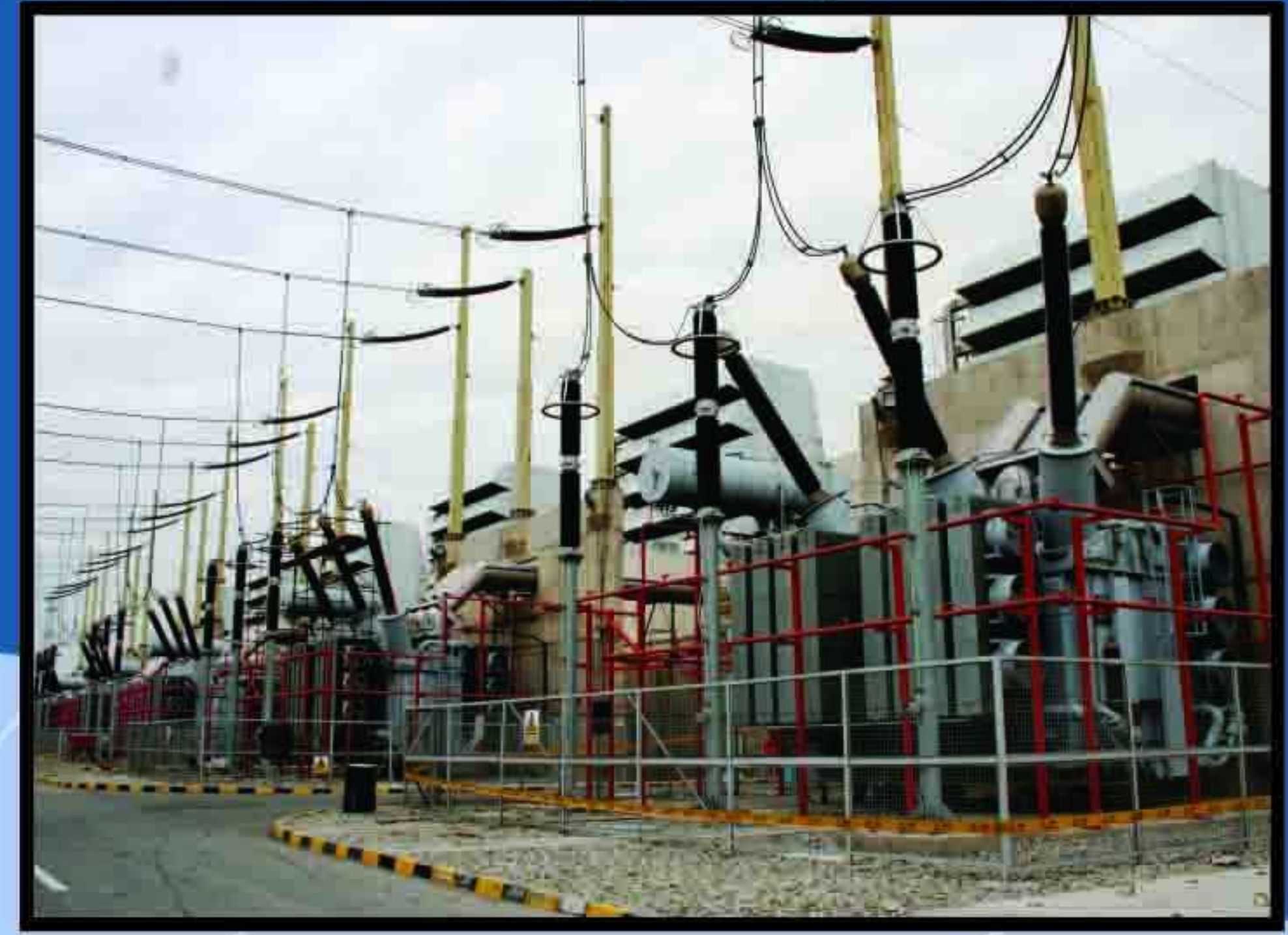
Damavand Power Plant 200 MVA - 15.7 / 420 kV
