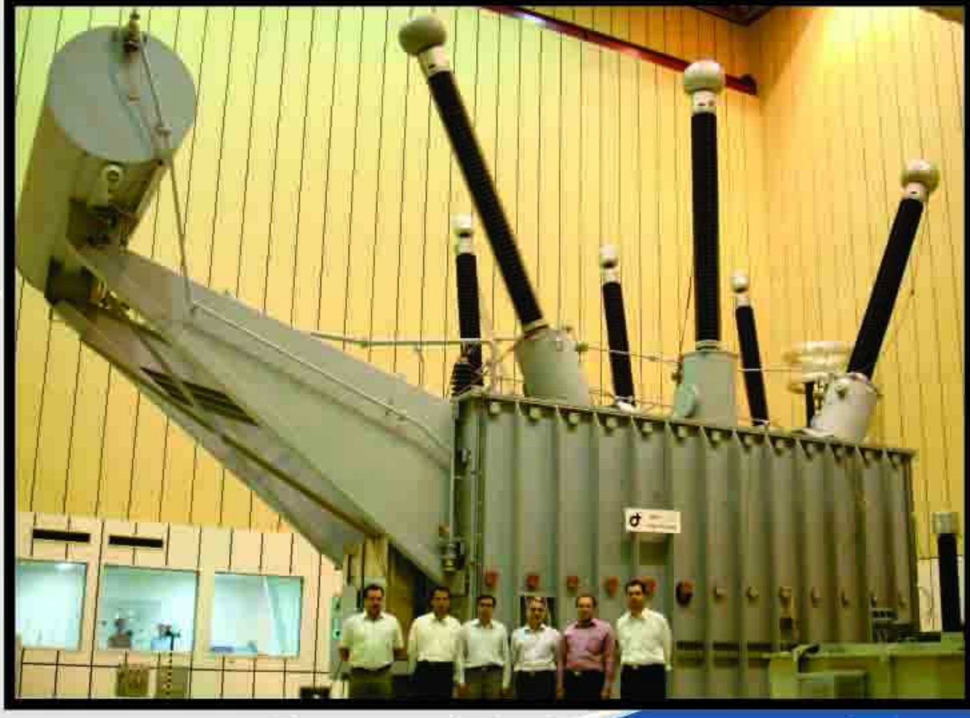
Power Transformer - Fars 315 MVA - 400 / 230 / 20 kV
