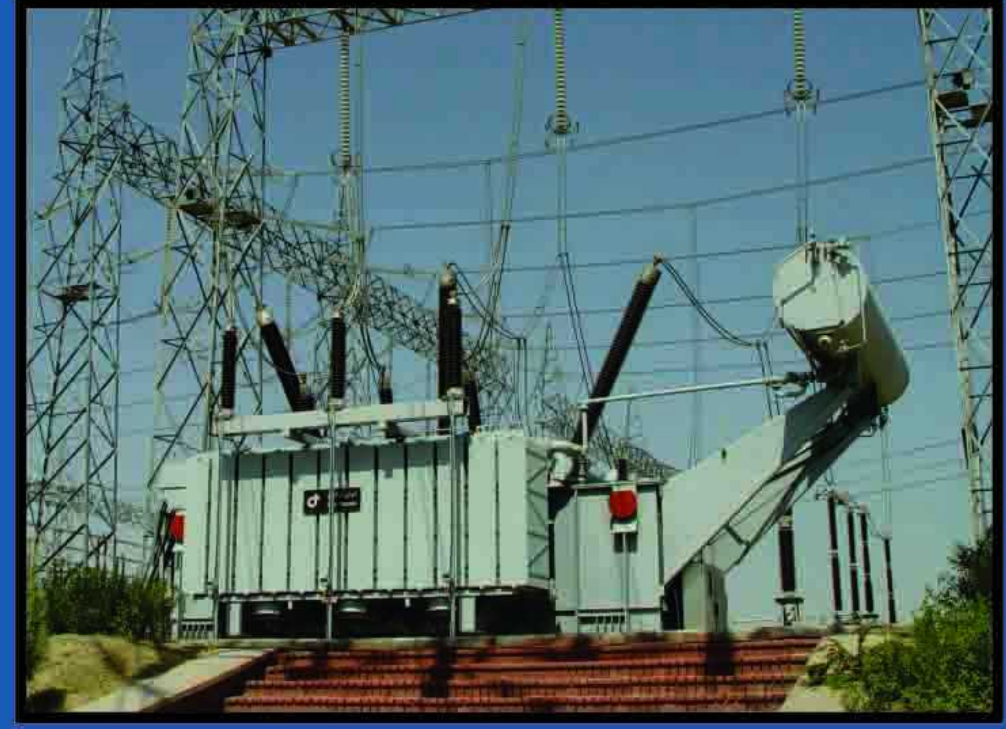
Tooss Substation 200 MVA - 400 / 230 / 20 kV
