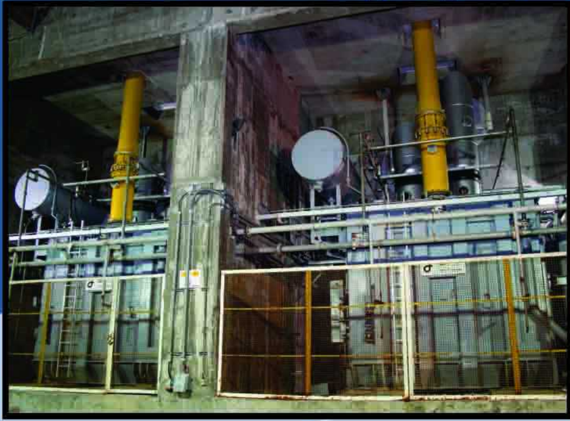
Karoon Hydro Power Plant 100 MVA - 15.7 / 420 kV
