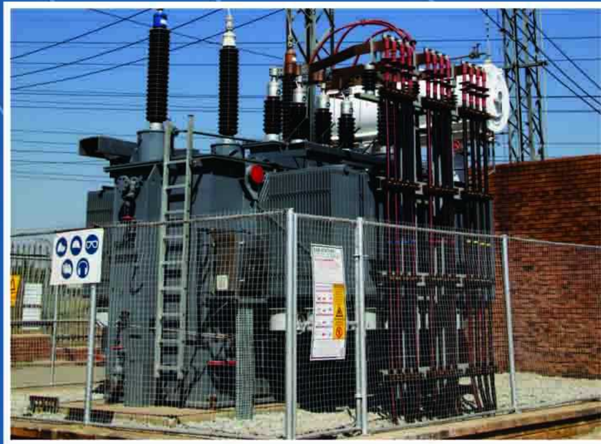
City Power - South Africa 45 MVA - 88 / 11 kV
