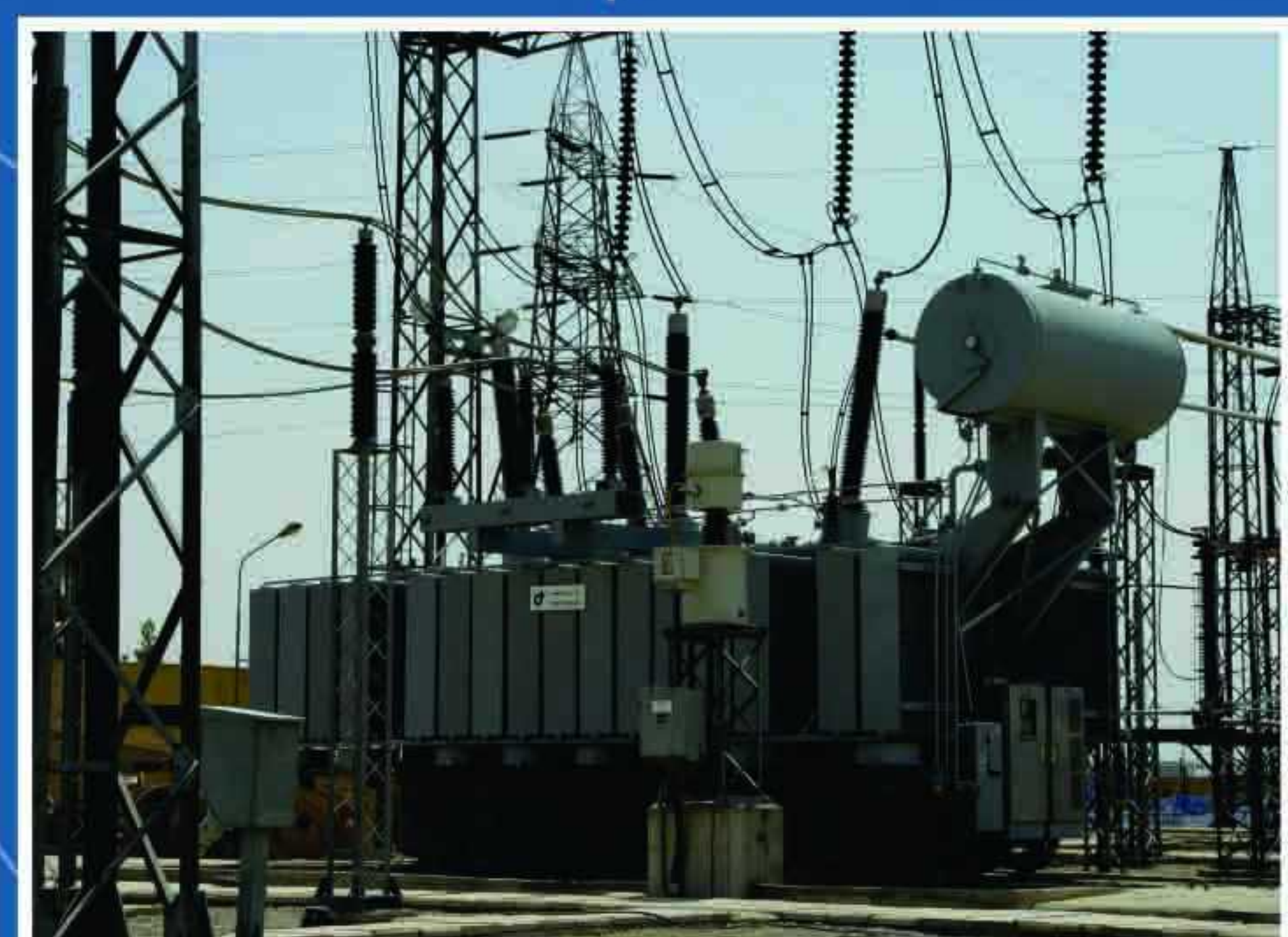
WAPDA Town Substation 40 MVA - 132 / 11.5 kV
