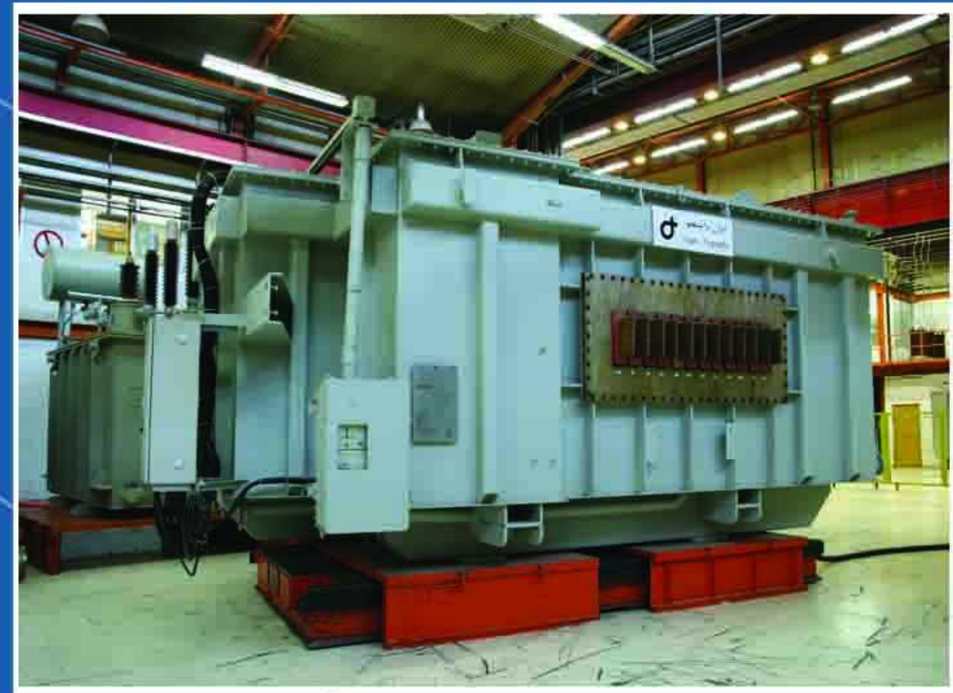
Furnace Transformer 30MVA -30.5KV/406V
