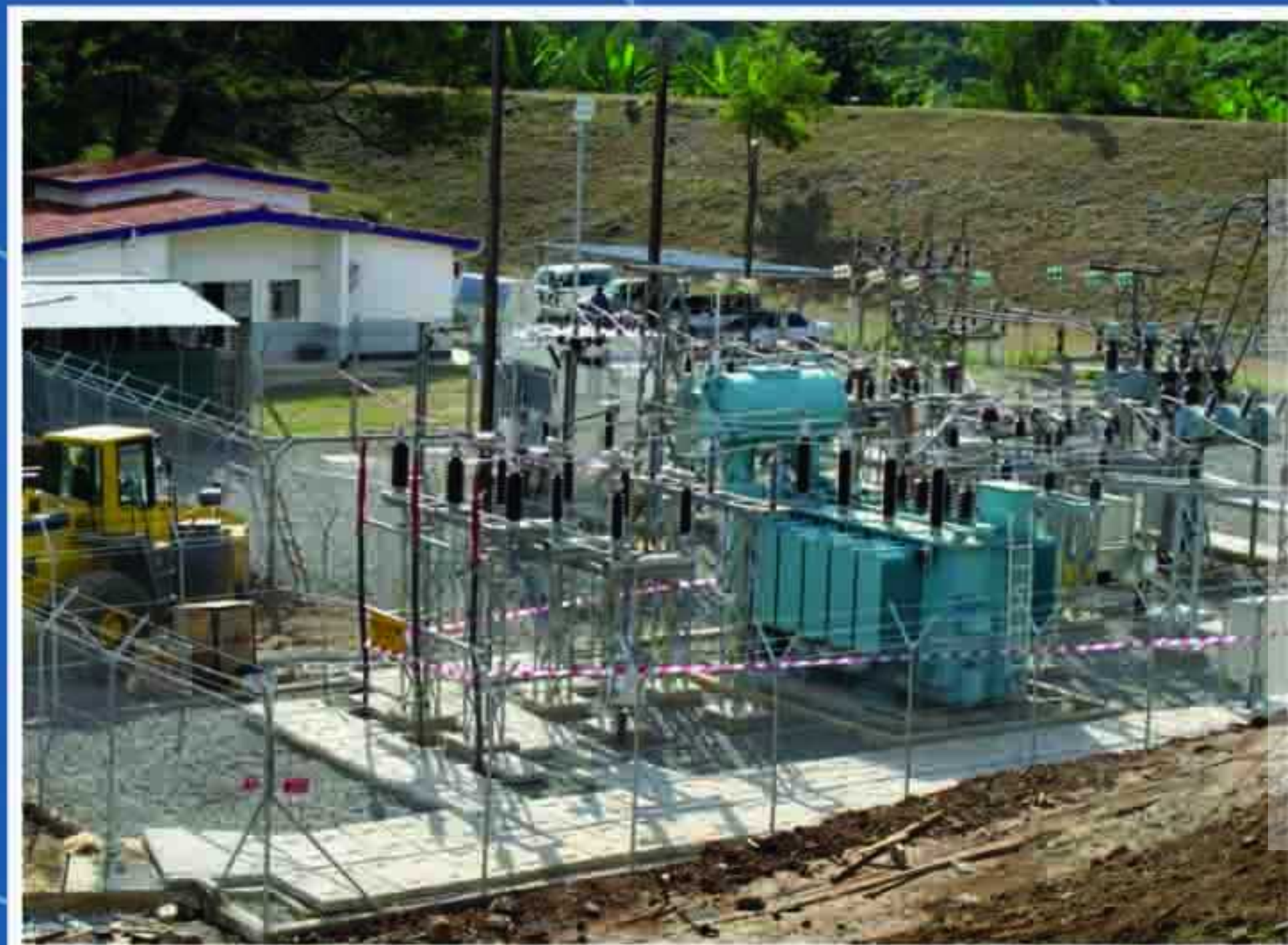
Tana Power Plant - Kenya 32 MVA - 71 / 11 kV
